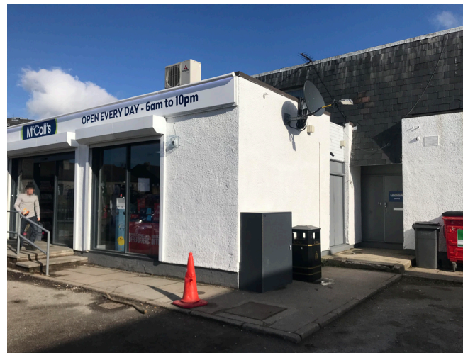
Temporary Accommodation above RS McColl's
